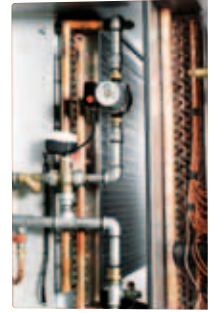
Built-in mixing circuit for water heating surface
